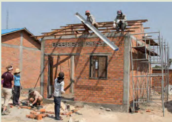
The roofing and rain gutters installation on Samon's home
